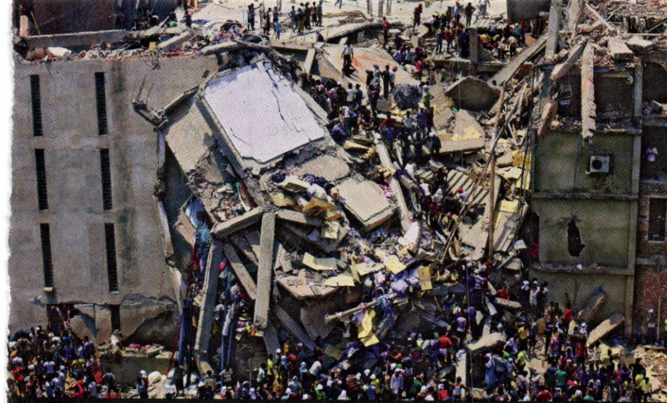
Bangladesh: Digging through the rubble of a clothing factory that collapsed in April, killing 1,127 workers
